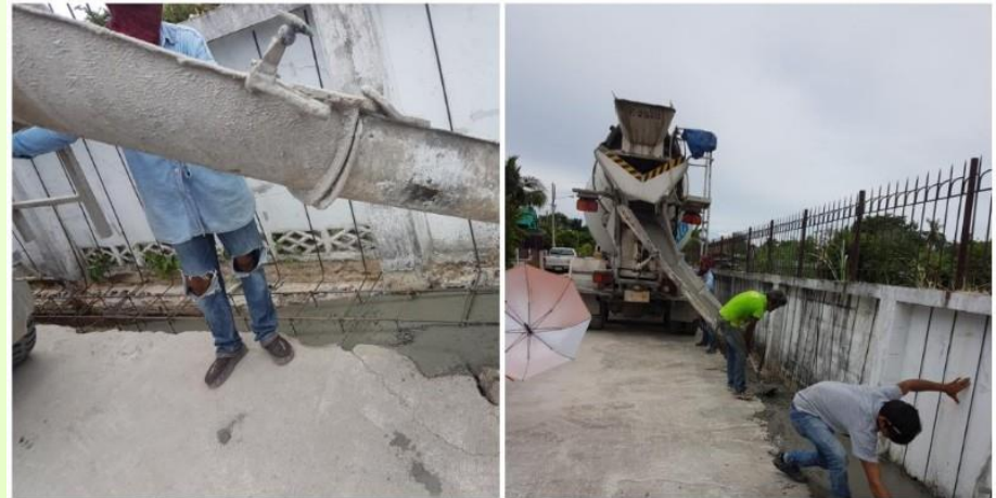
To make the strengthen foundations
